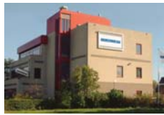
Mueller B.V. Sales Office Assen, The Netherlands
