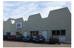
Mueller B.V. Service Facility Wesepe, The Netherlands
